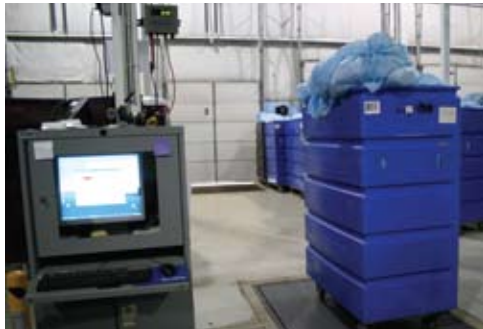
A computer monitor registers the weight of incoming soil goods. Goods are weighed on both the soil and clean sides of the plant.
