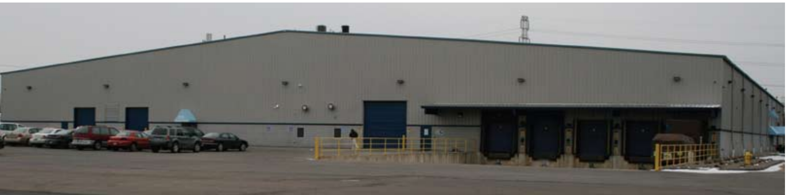
An exterior view of the Reino Linen plant, including loading bays at right.
