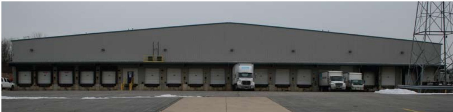
Another view of the loading area. Doors are numbered and customer names are written on the inside to help make sure the right goods get on the right truck.
